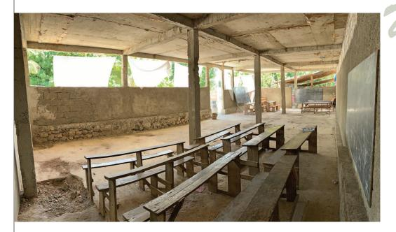
Work on the preschool building at Ti Goave has gone well, but it needs to be completed. The old tin roof which collapsed has been replaced with a solid concrete structure that will survive the severe weather that southern Haiti tends to get.
